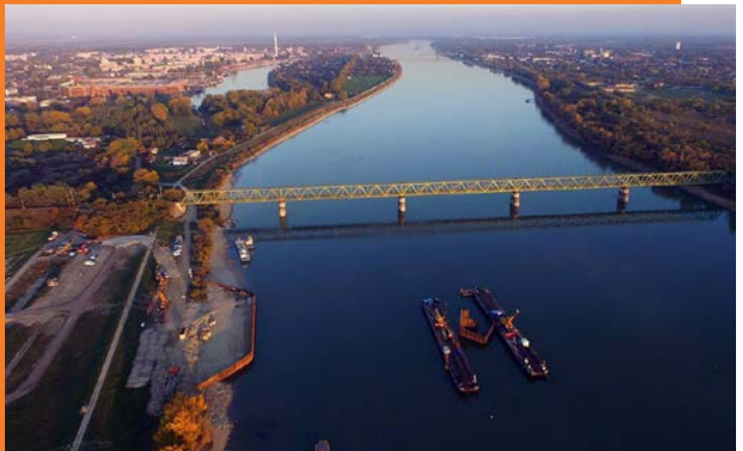
Cofferdams most Komarno
